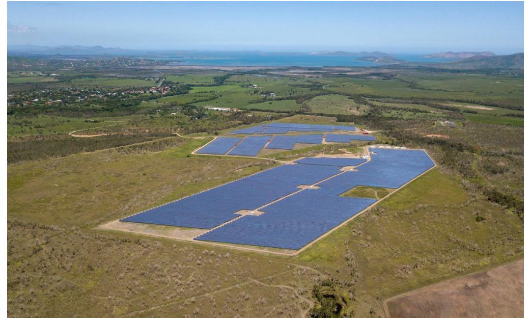
Figure: The Helio Boulouparis 2 Solar Park (16 MW, 10 MWh ESS).
