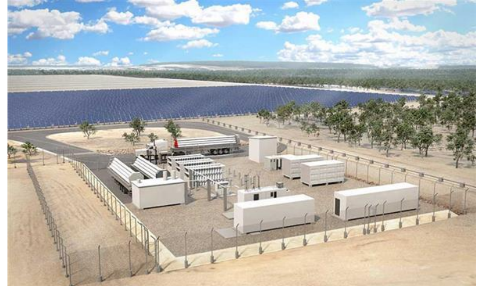
Figure: Kogan renewable hydrogen plant (1 MW electrolyser, 2 MW solar PV farm).
